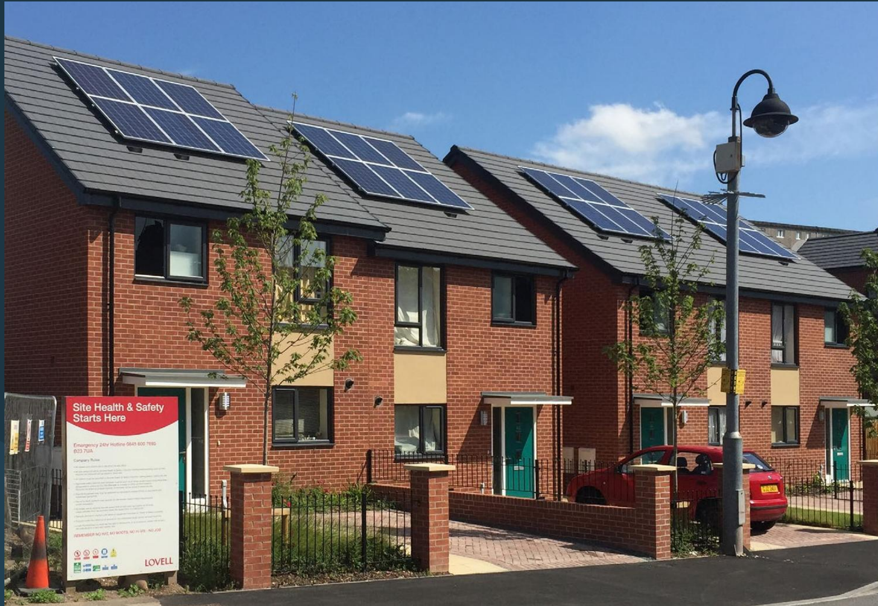
On-Roof Solar PV
