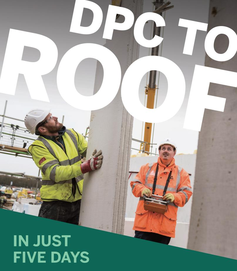
H+H UK Ltd can offer a fast build masonry alternative to both Timber Frame and aggregate. Our Vertical Wall Panels are erected onsite and can build a house shell from DPC to Roof in just five days.
