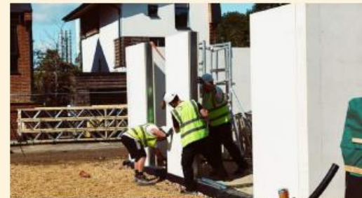
Project Etopia demonstration home, Watford, 2019, uses 'Hyper SIPS' high performing structural insulated panels, which include steel
