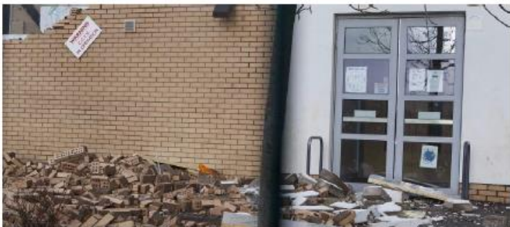
Image 4: Photograph taken at Oxfangs School of the gable wall after the collapse.
