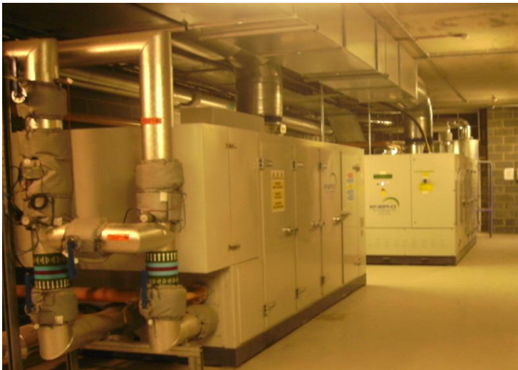
Combined Heat and Power unit - Lewisham
